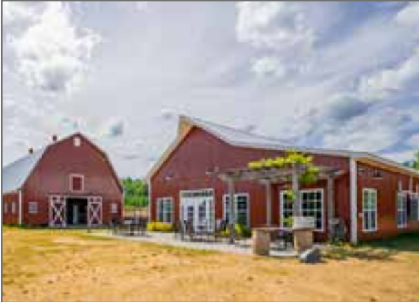
Building and other structures support agricultural and related business Uses
