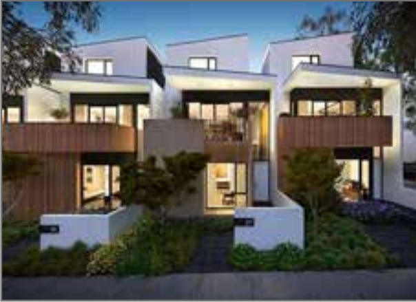
Row housing should have low front walls for privacy and Stepbacks can help reduce the perception of size
