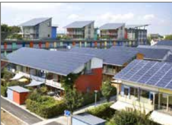
Sustainable Building options should be integrated into the design of new communities
