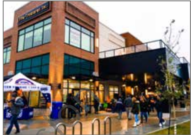
Buildings should be multiple Storeys with retail at Grade and commercial opportunities above, where possible.
